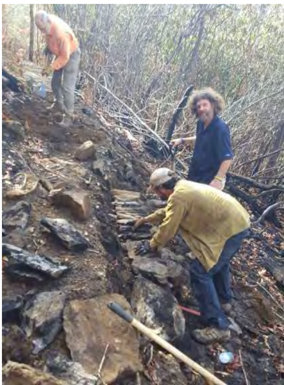
Repairing Sidehill Damage and Building Rock Retaining Wall
