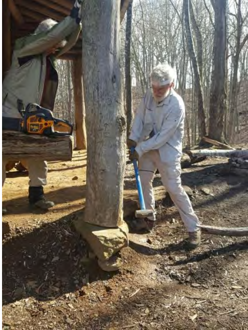
Photo- Dick Ketelle works at Brown Fork Gap Shelter
